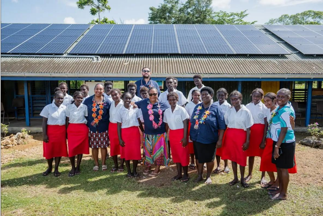
Caption 4: The AHC delegation, REnew representative and students and Principal of Goldie College standing in front of the solar panels.
